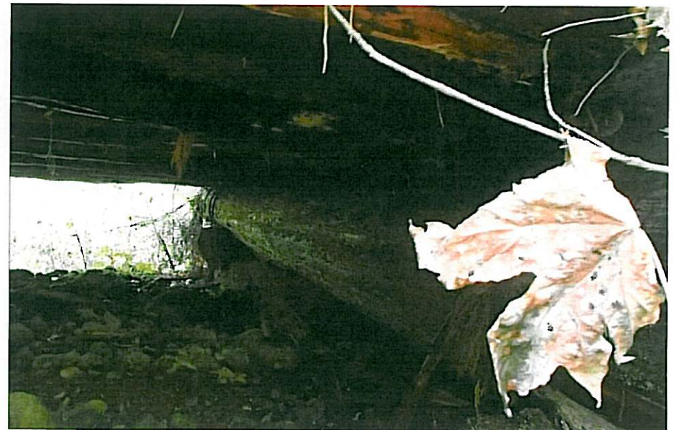
CK-2266 Right Abutment
